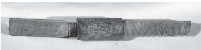
Plate 4 – Corrosion of Coupler
